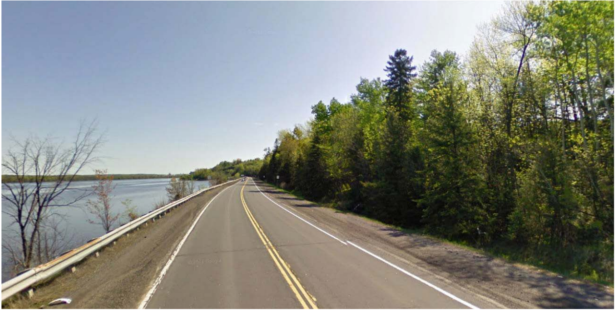
Photo # 5 – Highway 174 (Eastbound) near Proposed Collector Road
