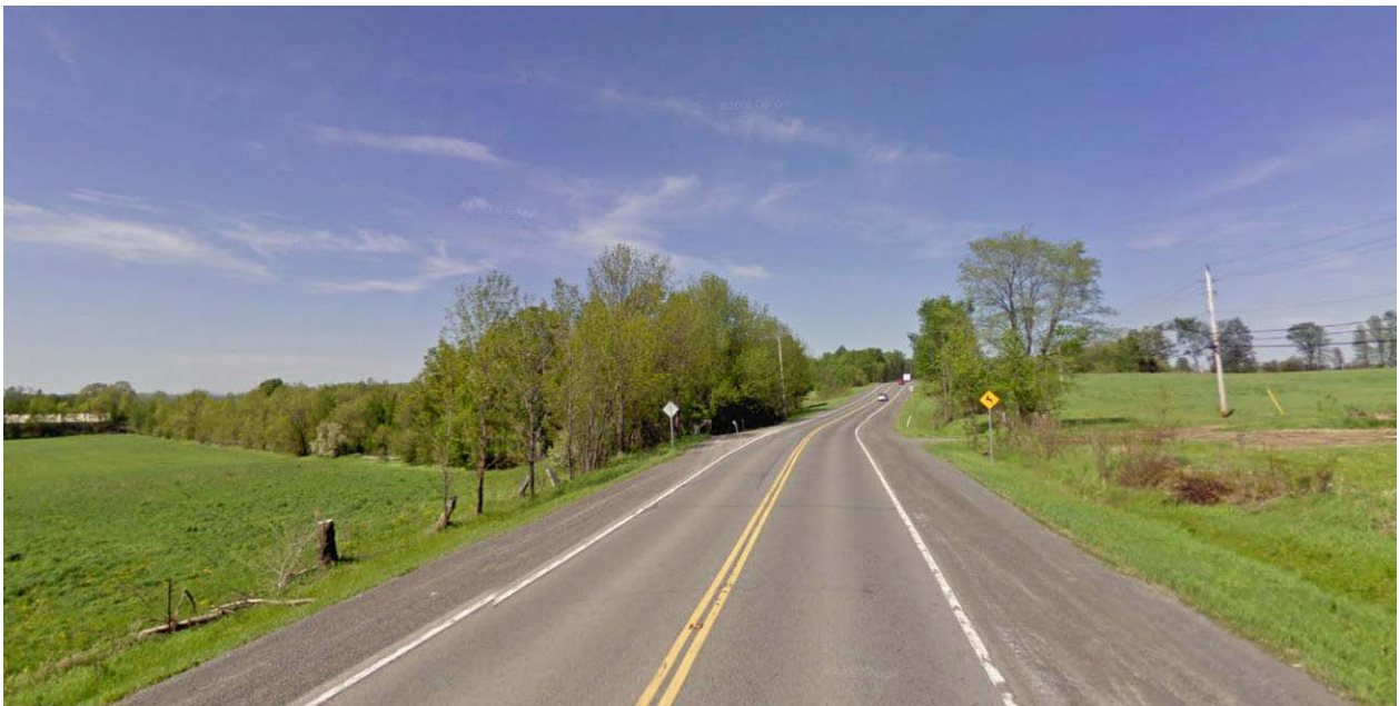
Photo # 6 – Old Montreal Road (Eastbound) near Proposed Collector Road
